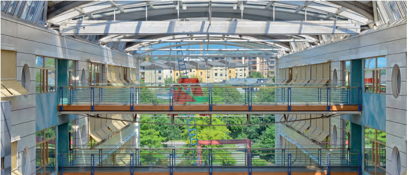
CFB-Fonds 150, Joseph-Bech-Building in Luxemburg
