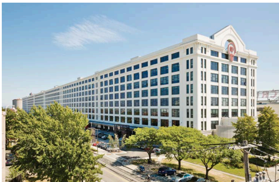
Innovation and Design Building 17, 19, 21, 23, 25 Drydock Avenue Boston, Massachusetts, USA Mietflächen in qm: 125.737 Vermietungsstand: 91%
